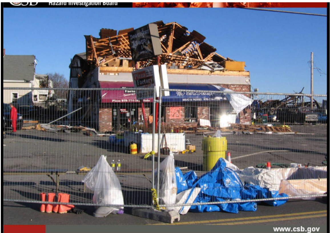
Businesses were damaged because of the blast
