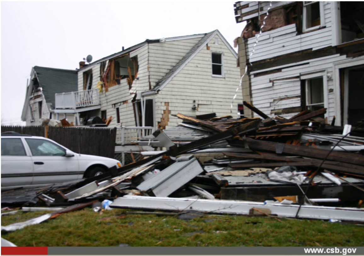
Severe structural damage to nearby houses occurred because of the blast
