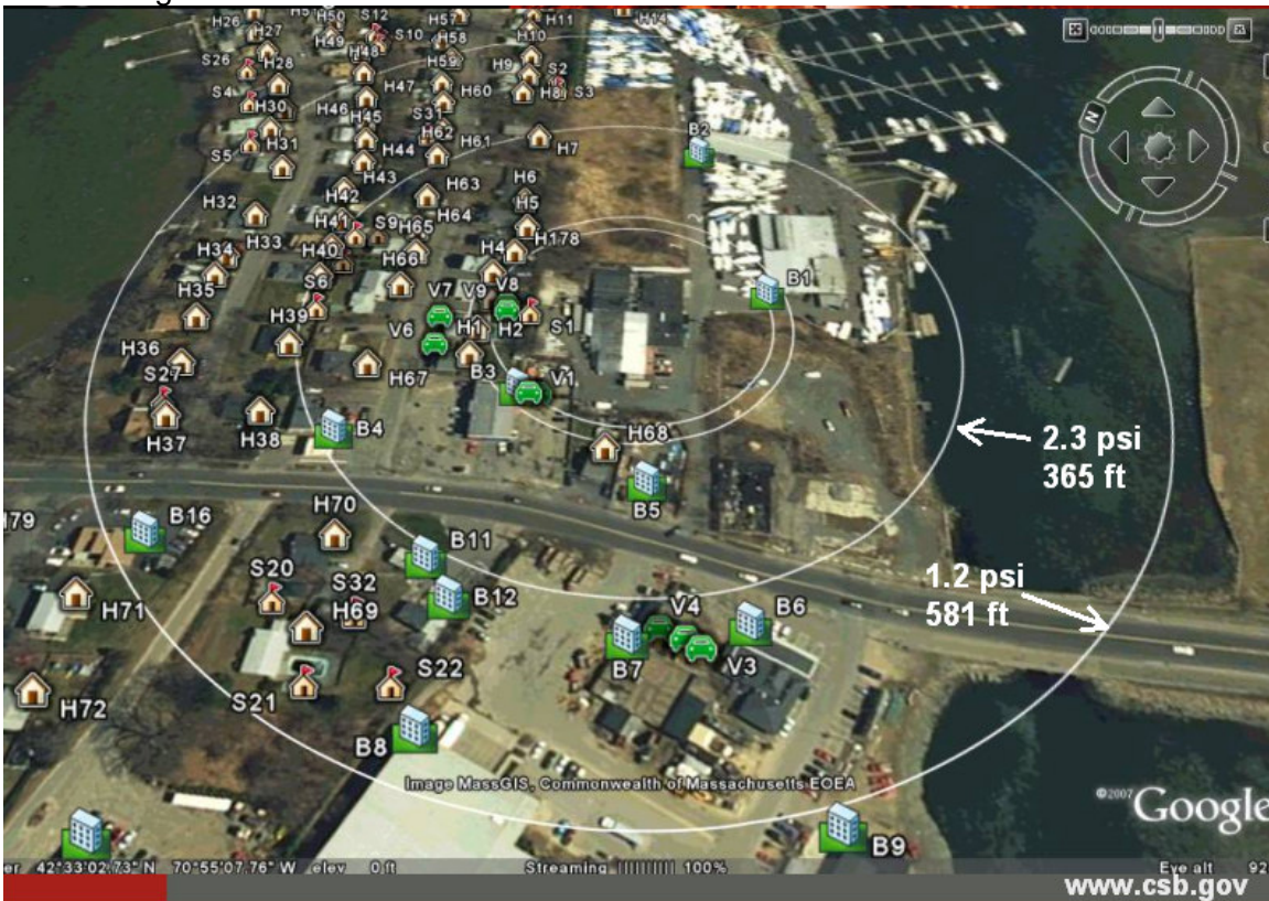
A key part of the CSB investigation was to map damage assessment as a function of distance from “ground zero” and relate to peak blast overpressure. The above image is
