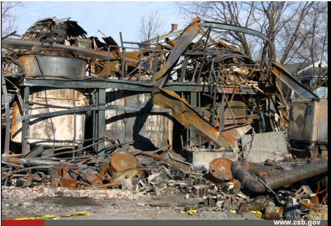
The CSB examined what was left of equipment at the facility. Note proximity of nearby house at right.
